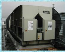
EcoMESH in front of the heat rejection coil provides a self-cleaning filter which in return keeps the coil clean. This is achieved by the mechanical design of the double mesh concept as well as jet water spray over the mesh against the air stream. By keeping the coil clean the overall system efficiency could be improved as much as 3~5%.
